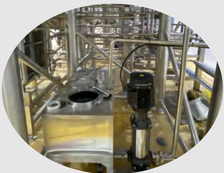
Condensate Tank System
