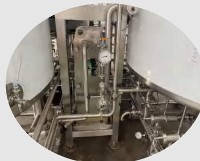
Plate Heating Exchanger
