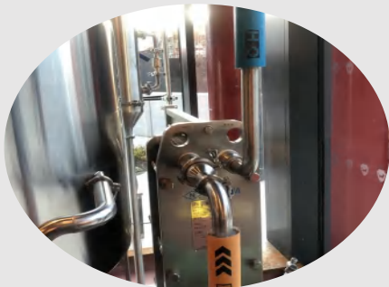
Plate Heating Exchanger
