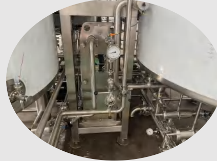
Plate Heating Exchanger
