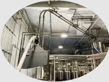
Screw Conveyor System
